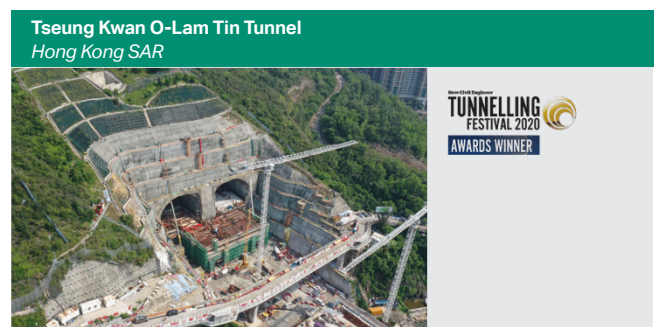
Large-scale semi-caverns as part of road tunnels
