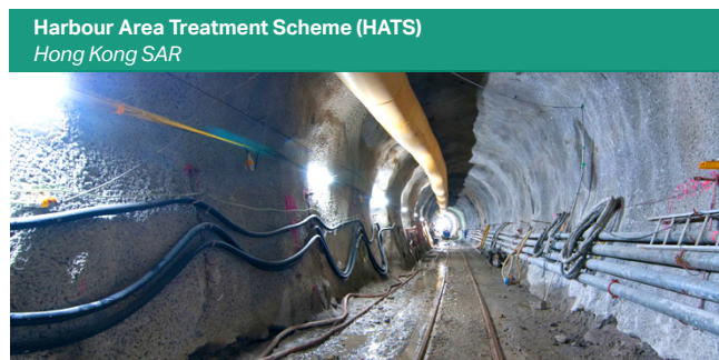
Deepest sub-sea tunnel (160 m below sea) in Hong Kong SAR
