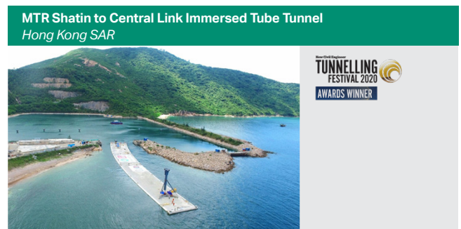
1.7-km-long railway immersed tube tunnel
