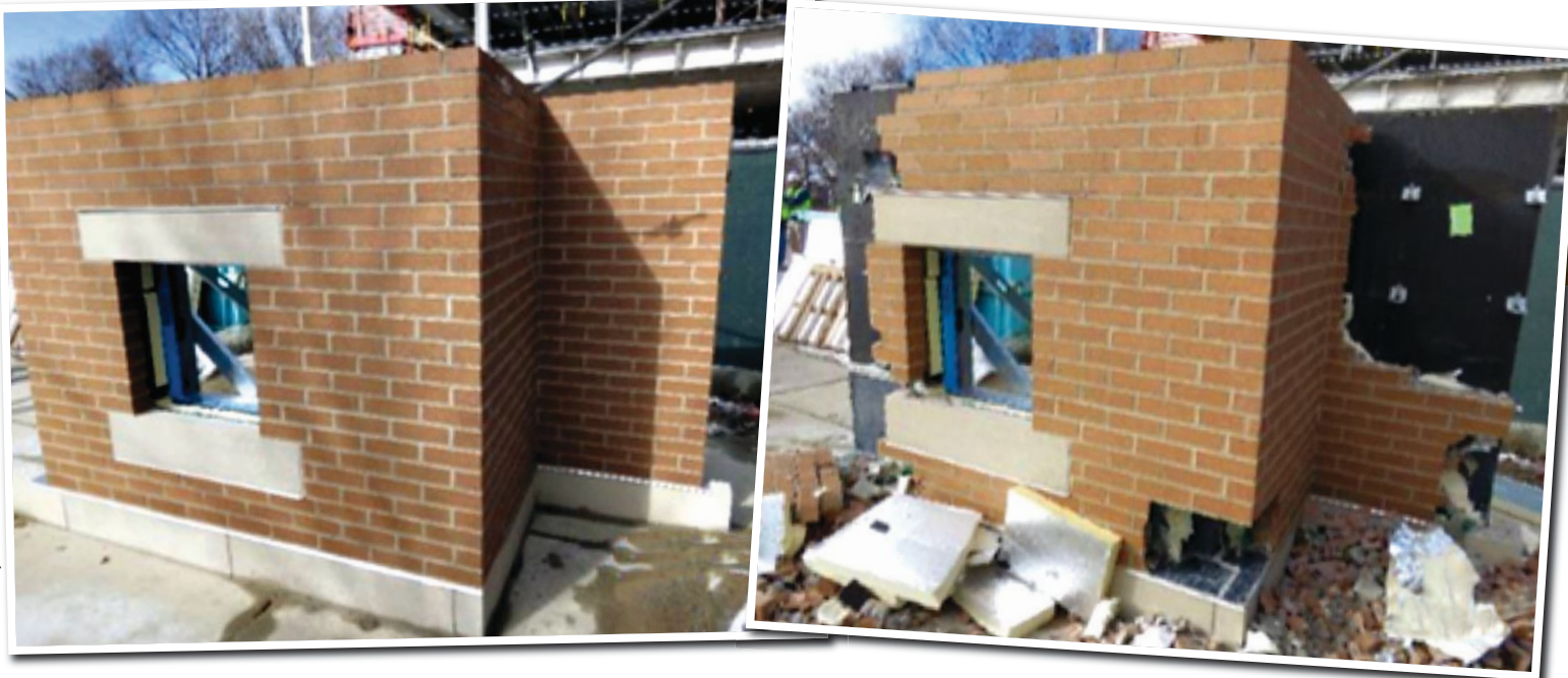
Photos Courtesy of Pepper Construction
